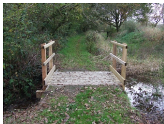
Replacement Dunsdon Nature Reserve footbridge
