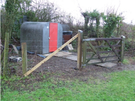
Refurbished store and fencing
