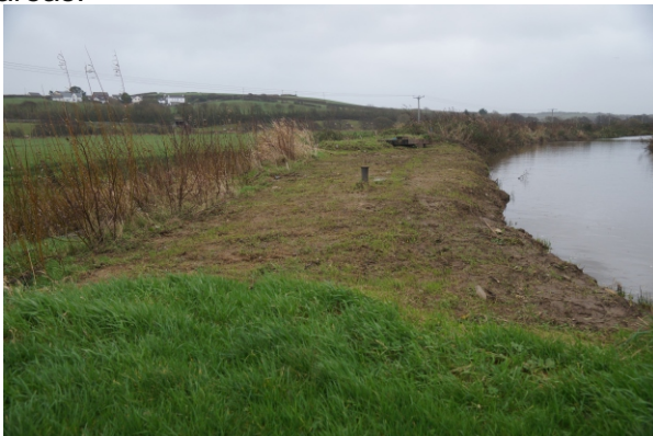
Current temporary spillway
