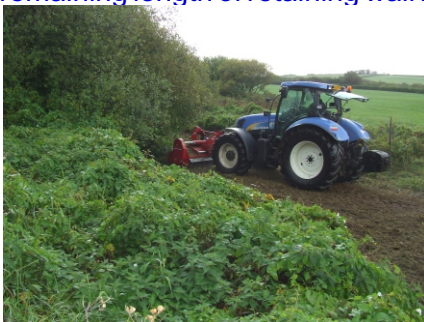
Initial mechanical clearing
