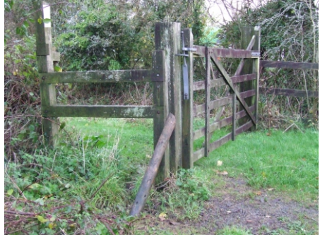
Repaired gate and removed stile
